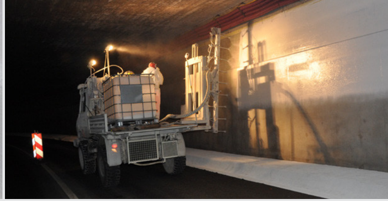
Picture left: The Jordiguhittini gallery in Simplon, Switzerland is protected with Emcephob HPC surface coating in RAL 9010. Picture right: Automated coating work in the Schallbett gallery by Trauffer AG, Brienz.
