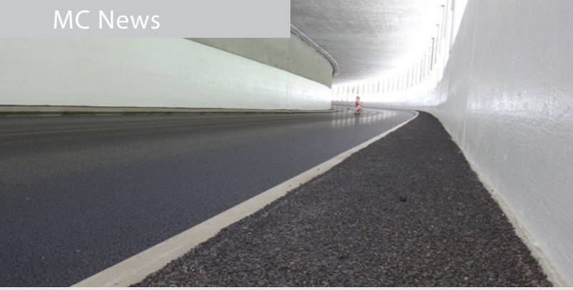
Picture left: The Jordiguhittini gallery in Simplon, Switzerland is protected with Emcephob HPC surface coating in RAL 9010. Picture right: Automated coating work in the Schallbett gallery by Trauffer AG, Brienz.
